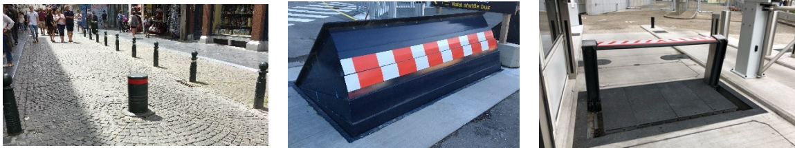
Figure 41. Typical active barriers.
