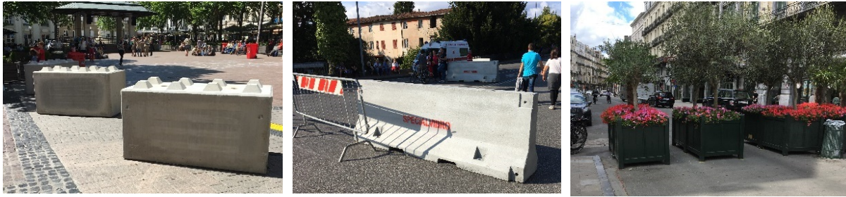
Figure 37. Typical temporary protective barriers.
