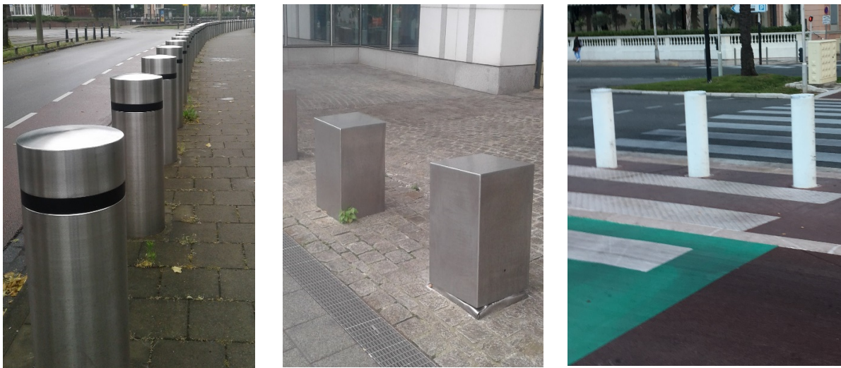
Figure 36. Typical protective bollards.
