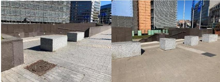
Figure 22: Granite-covered benches protecting the Berlaymont esplanade staircases
